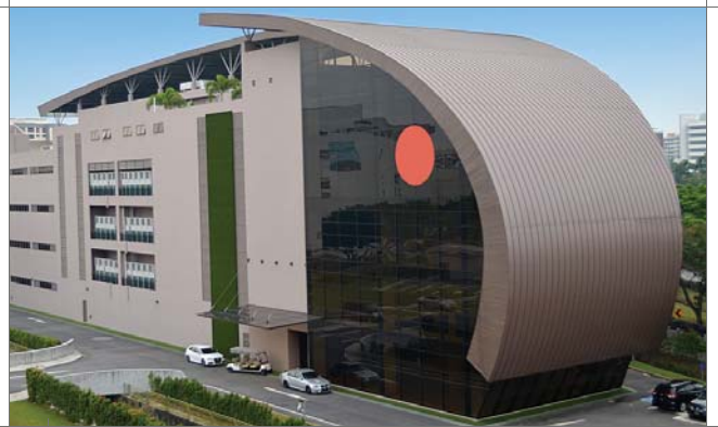
Industrial Building, Singapore
